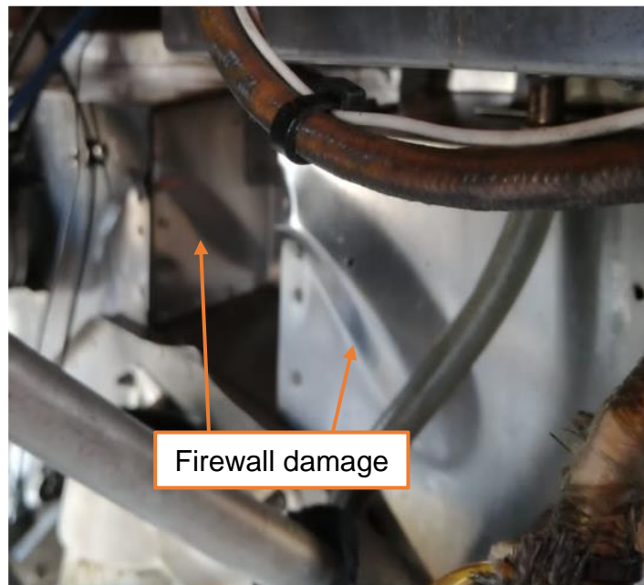
Figure 2: Damage to the firewall. (Source: Operator)
