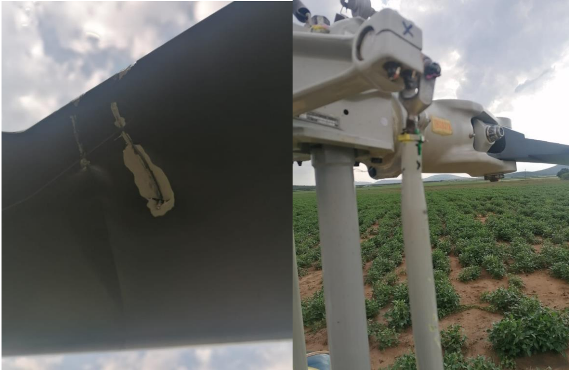
Figure 2: Damage to the main rotor blade and the bent pitch link. (Source: AME)
