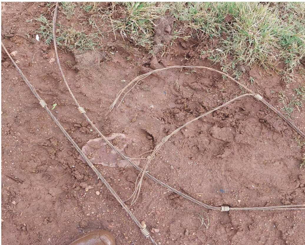
Figure 6: The severed cables.
