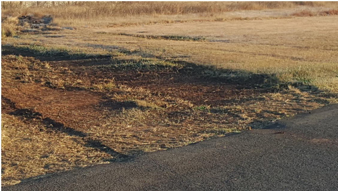
Figure 2: Water runoff point. (Source: Pilot)
