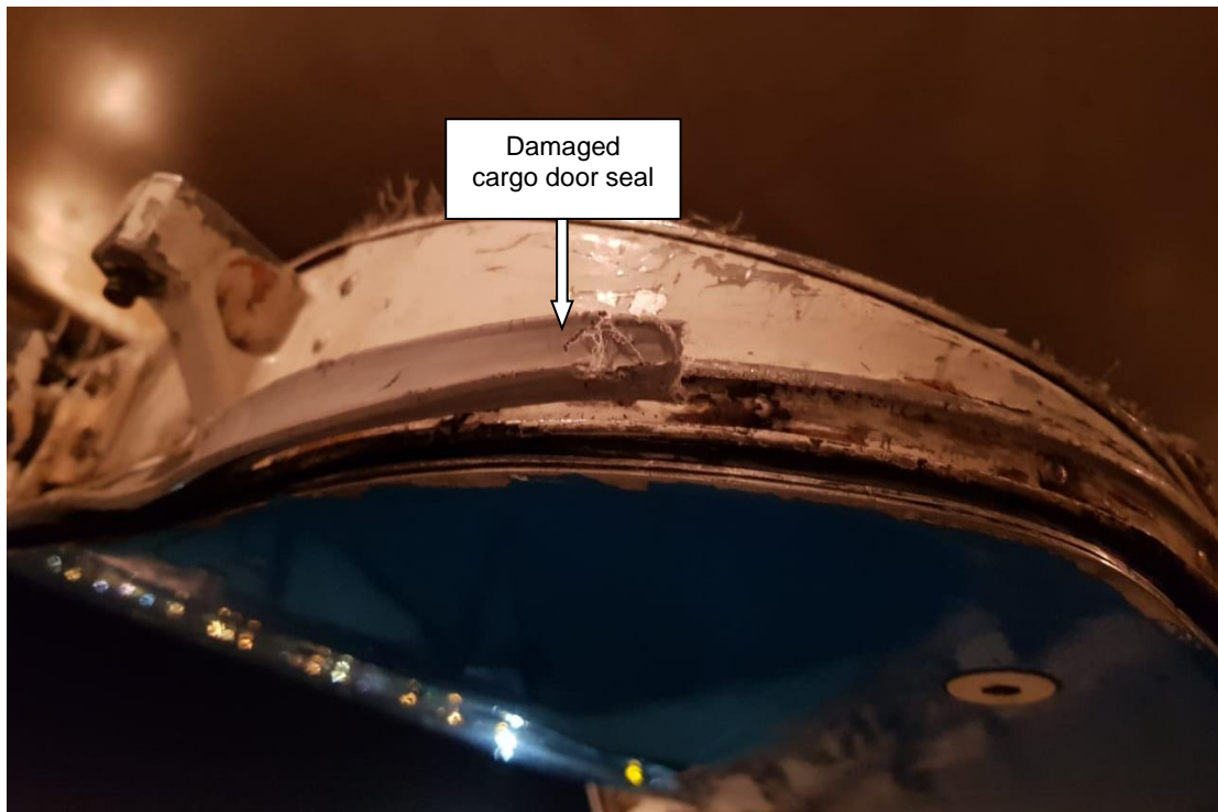
Figure 9: A section of the damaged aft cargo door pressure seal.
