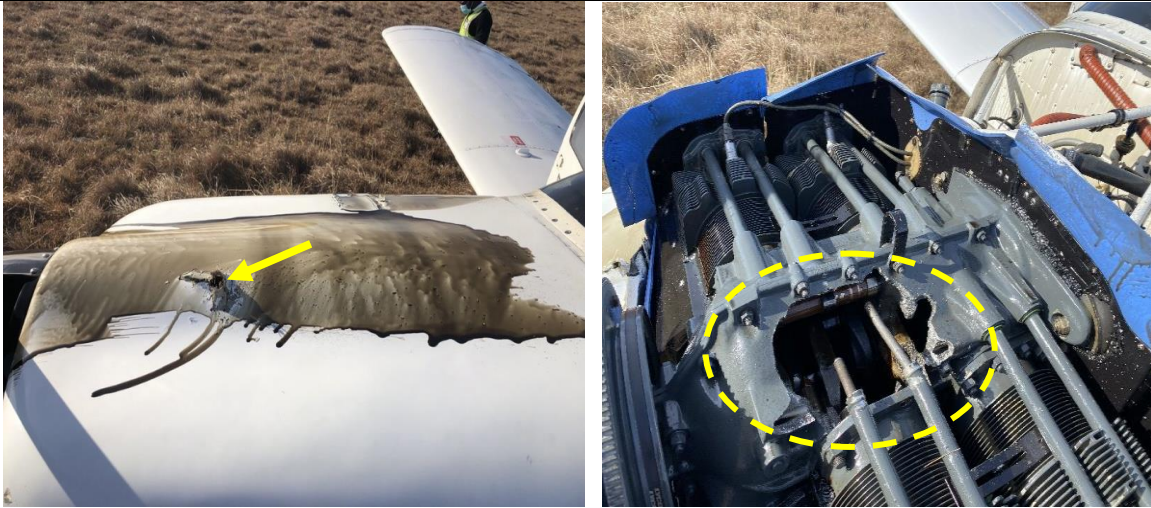
Figures 2 and 3: Damage on the engine top cowling (left picture). Damage on the upper left part of the crankcase (right picture). (Source: Operator)
