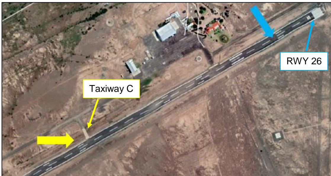
Figure 1: Aerial view of FABW. The blue arrow shows touchdown point; the yellow arrow shows the point where aircraft came to rest. (Source: Google Earth)
