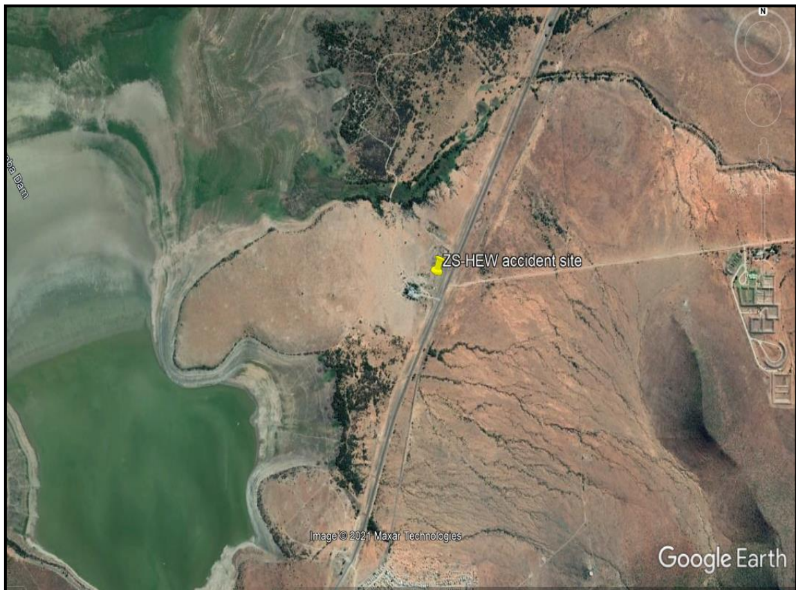
Figure 1: A view of the incident site. (Source: Google Earth)
