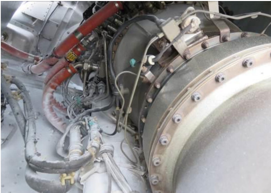
Figure 8: The engine nacelle with evidence of fire extinguisher contents having been discharged
