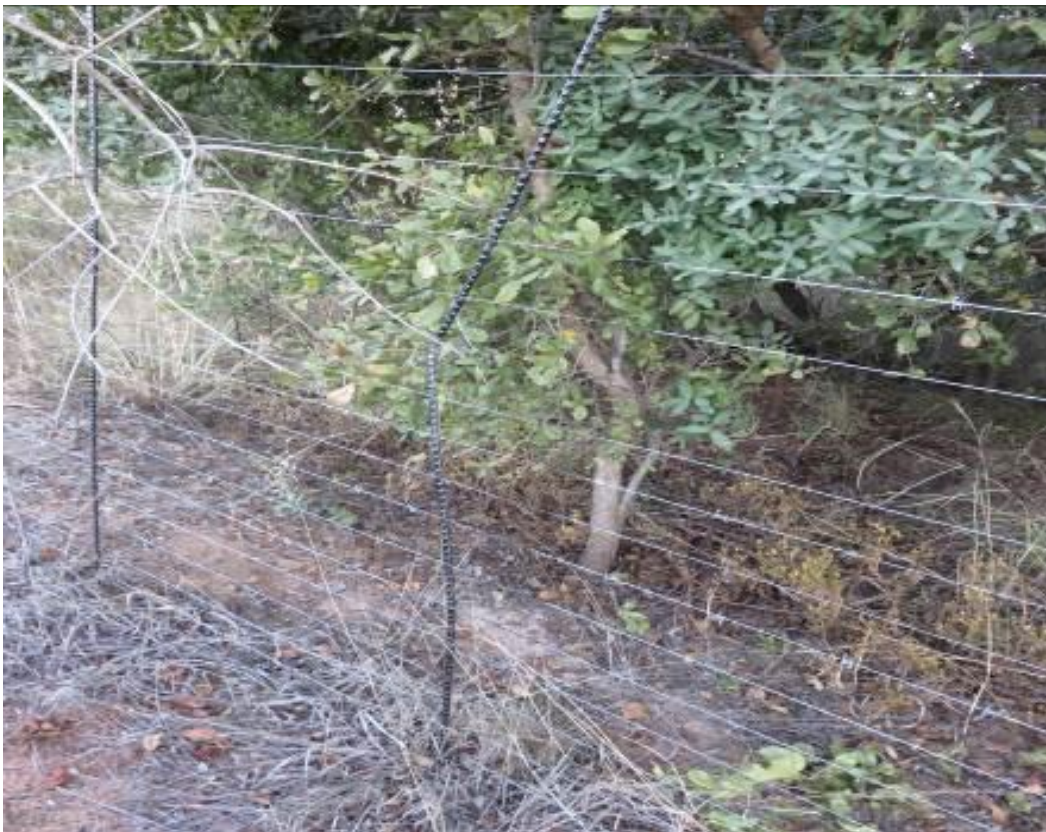
Figure 3: Damage to the steel rod and fence.
