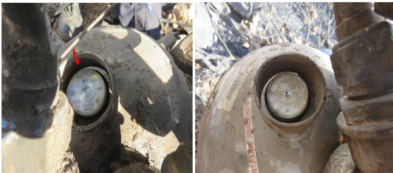
Figure 14: The condition of the fire extinguisher bottles as found at the accident site. The gauge on the left-hand side reads '500psi' and the other gauge was unreadable and heavy, indicating that it contained the fire-extinguishing agent that was never used. This was an indication that both bottles were never discharged. In addition, two fire-extinguishing system discharge switches were in the 'off' and guarded position (refer to Figure 12 above), confirming that the crew neither activated nor discharged either of the fire-extinguishing systems.
