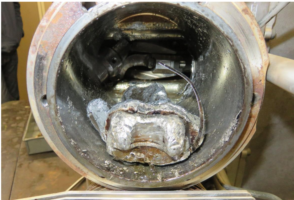
Figure 5: Visible fragments within the No. 4 cylinder are fragments of the piston and a deformed conrod
