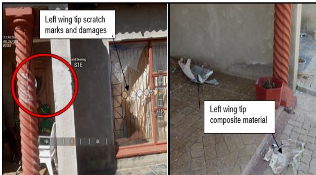
Figures 8 and 9: Scratch marks of the left-wing tip on the pillar and the damaged window.
