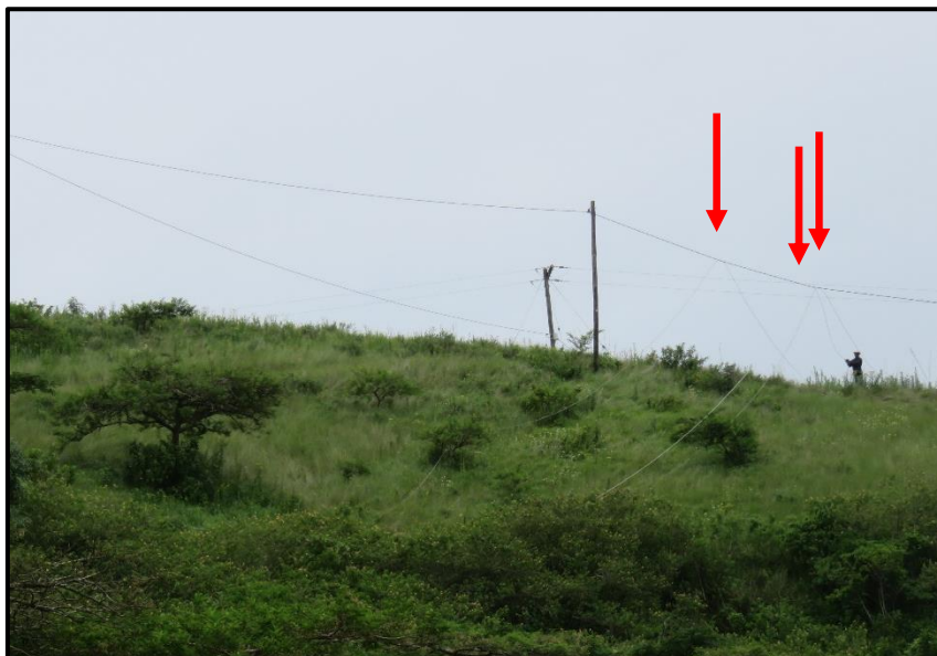
Figure 3: Damaged high-tension wire.
