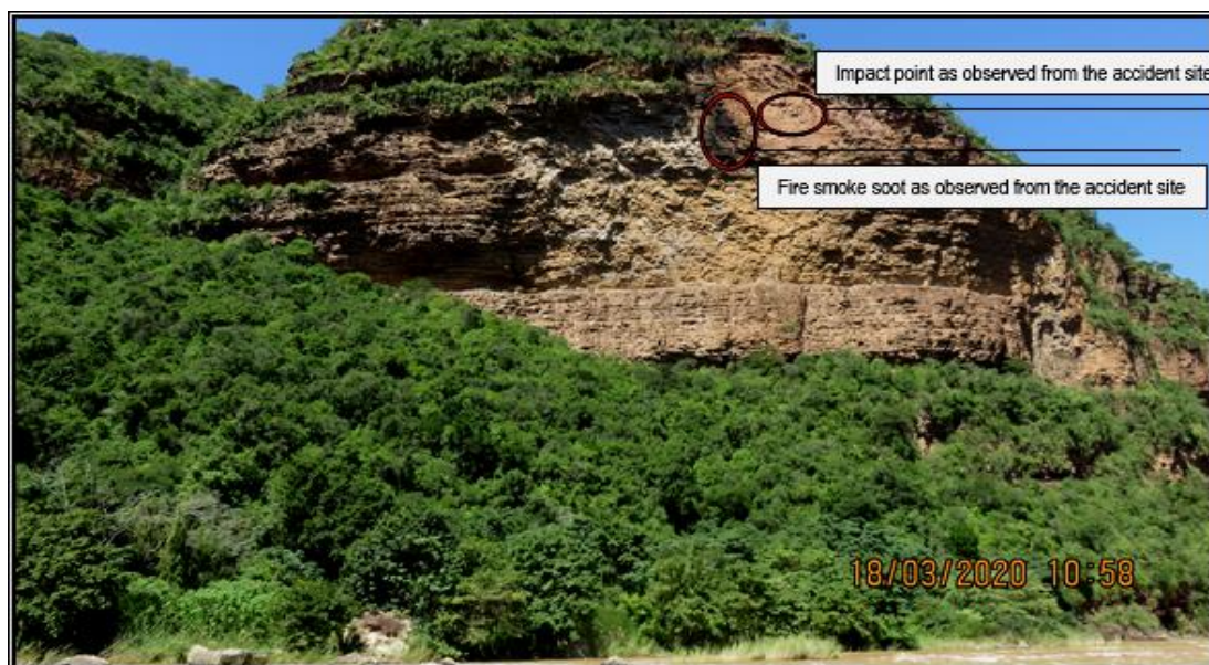
Figure 9: Soot left by an explosion at the place of impact.
