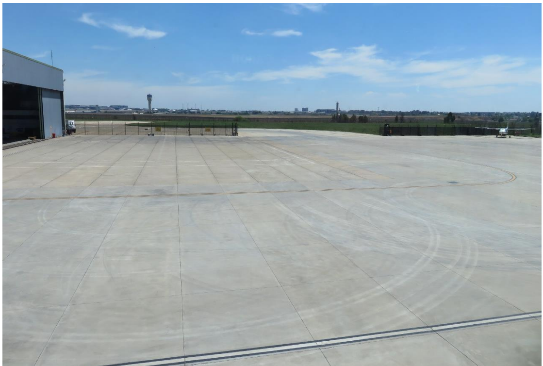
Figure 19: The FBO apron area. The picture was taken from the FBO operations centre.
