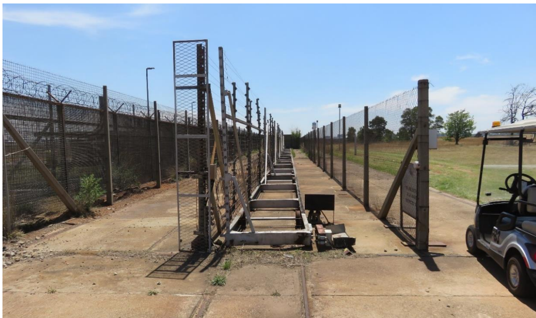
Figure 10: The Denel Campus gate stationary in the fully open position.
