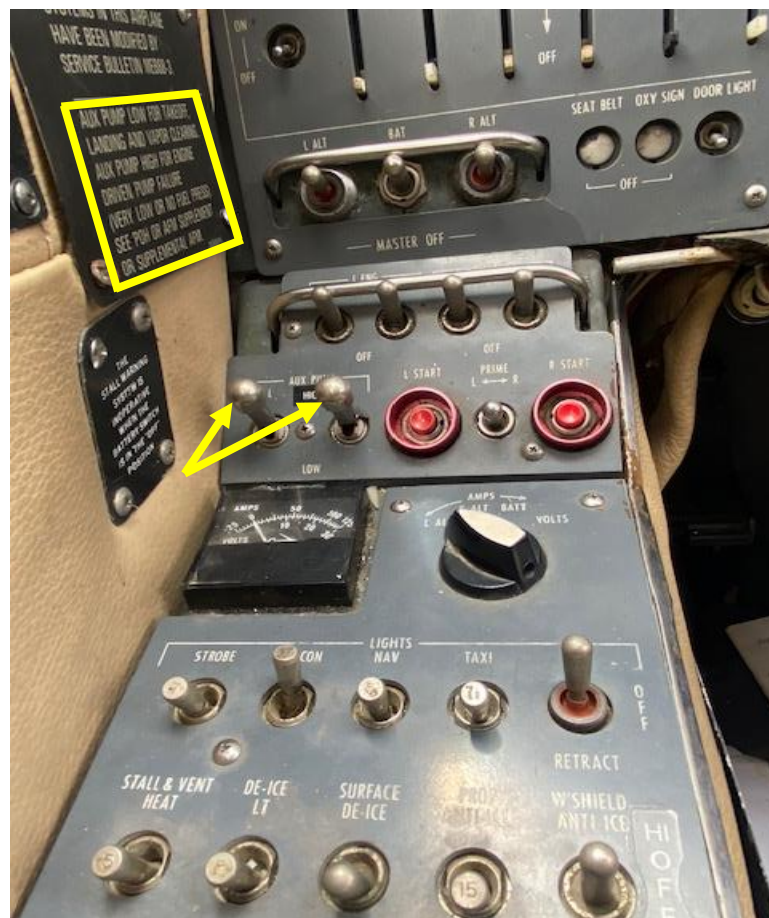
Figures 11/12: View of the auxiliary pumps in a HIGH mode setting. There is a placard (yellow window above) installed on the left pilot side panel indicating AUX PUMP HIGH FOR ENGINE DRIVEN PUMP FAILURE (VERY LOW OR NO FUEL PRESSURE).
