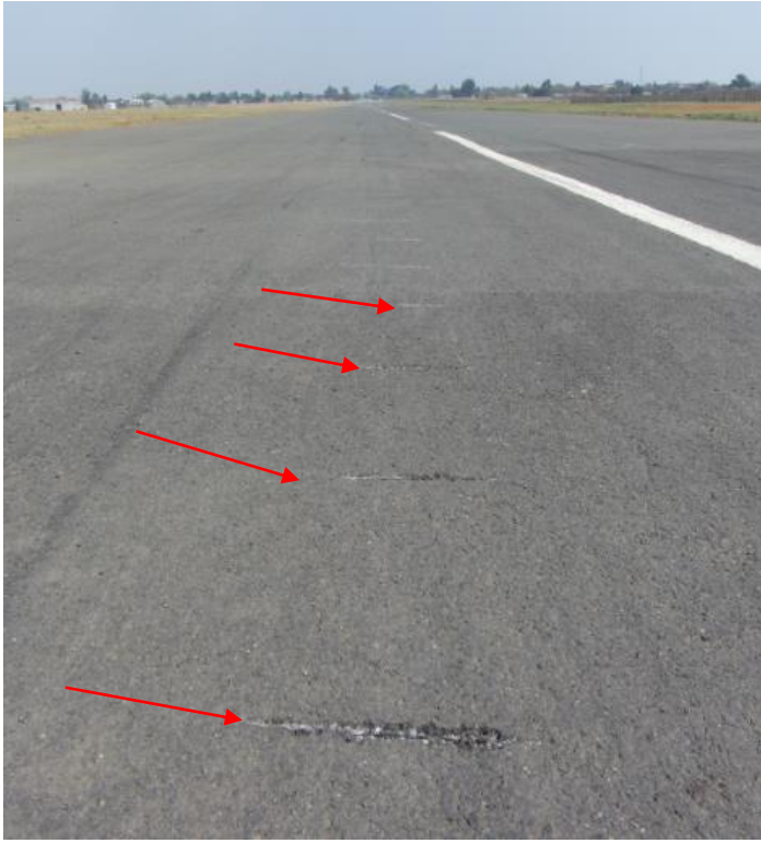
Figures 4 and 5: Arrows showing left- and right-side propeller tip marks on the asphalt runway.
