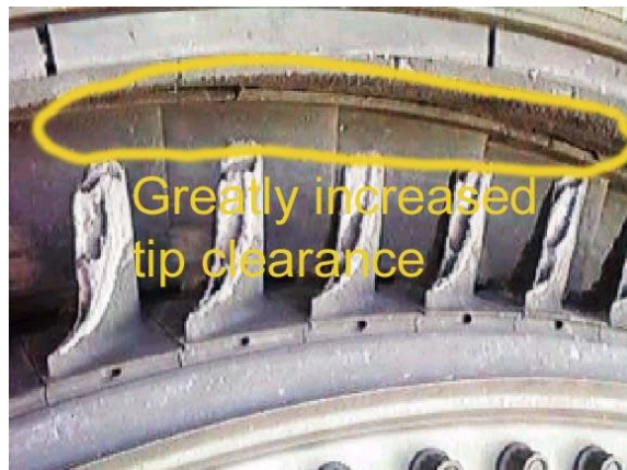
Figure 24. Increased tip clearance caused by overheat
