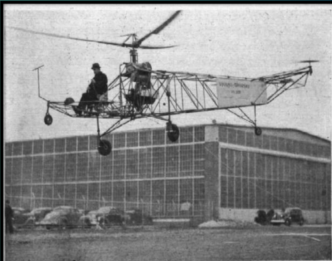
TESTING THE CONTROLS. Mr. Igor Sikorsky makes the first ascent on his new helicopter. Note that the machine is "tethered." Subsequently several free flights were made.
