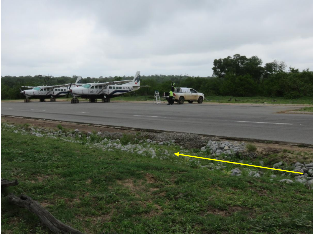
Figure 4: The water drainage ditch next to the runway edge apron area.
