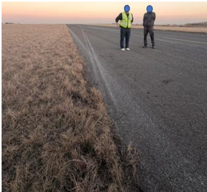
Figure 2: The aircraft's skid marks on the runway. (Source: Operator)
